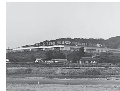
The Hiroshima Plant, a dedicated radio factory (1967)
