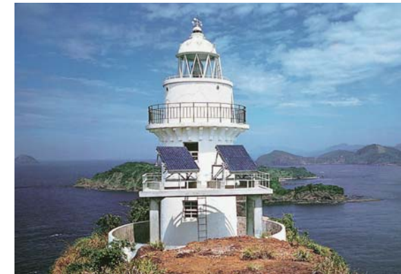
The Ogami Island Lighthouse is powered by Sharp solar (photo courtesy of Japan Coast Guard)
